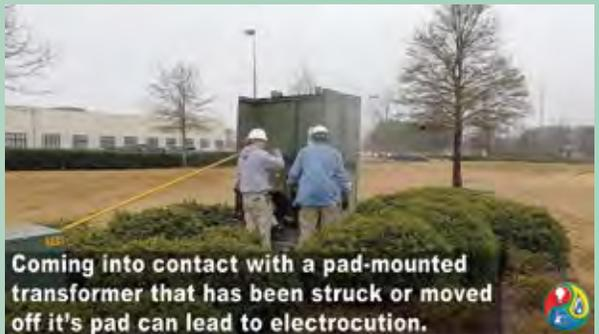
**Coming into contact with a pad-mounted transformer that has been struck or moved off it's pad can lead to electrocution.**
