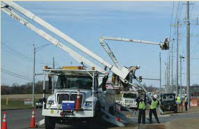
Electric crews are currently working along County Line Road preparing delivery lines for the 46kV portion of the new substation built to feed from TVA's County Line Delivery Point. The 12 kV portion of the substation is already online.
