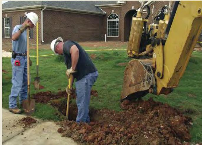
Utility crews locate gas service lines manually, using shovels instead of backhoes, to avoid pipe damage when within 18 inches of the pipe. Not only does this action save money, but it may save lives.
