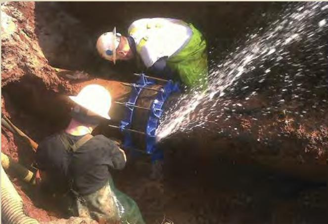
Water Operations crew members repair a leak on an 18-inch water main on Ninth Avenue.
